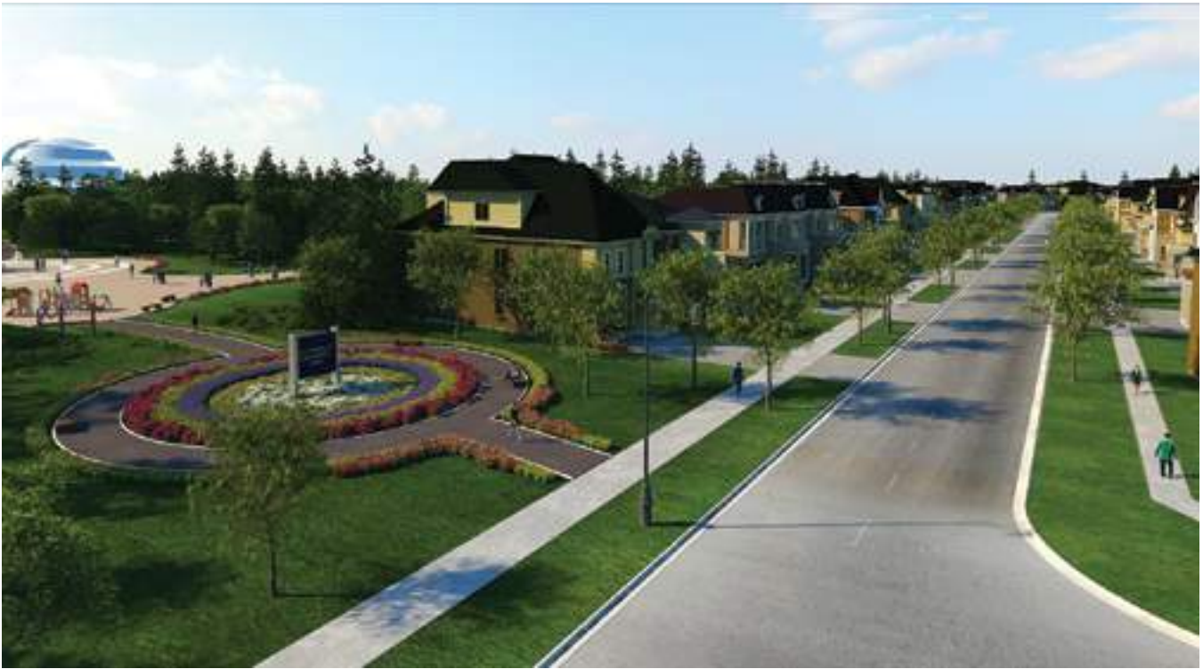
East Entrance on David Dunlap Boulevard
